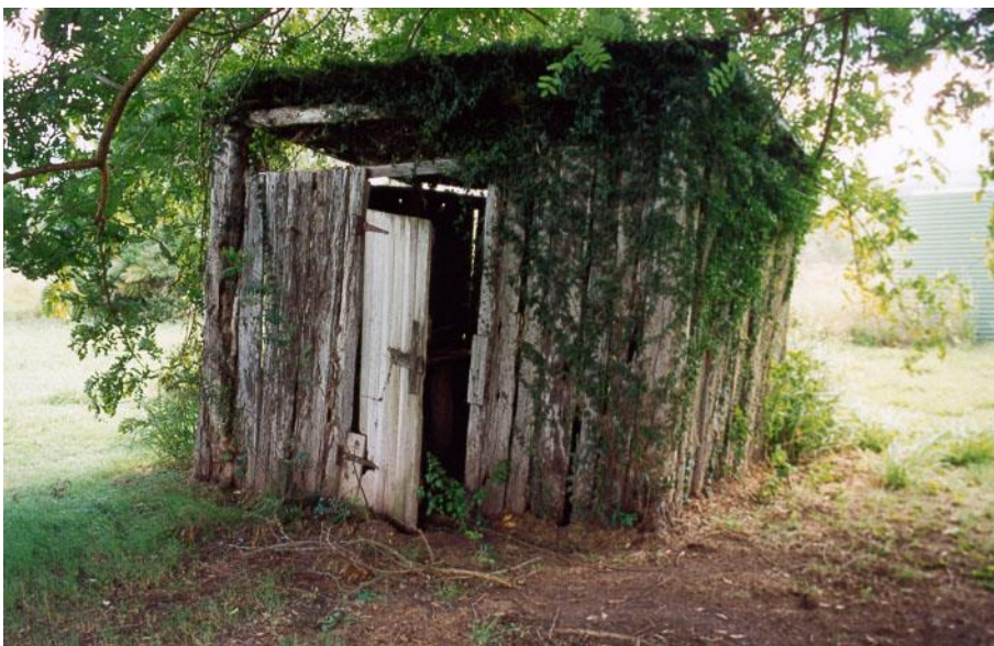
Former cream shed
