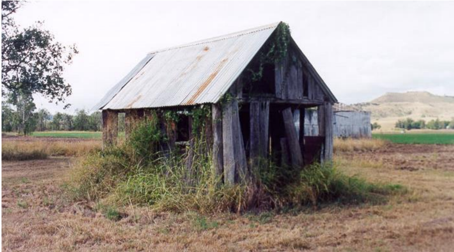
Former buggy shed
